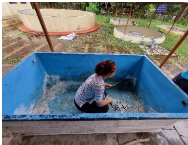
Fig 2: Roughly cleaning of tank
